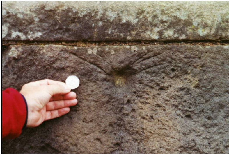
Figure 127: Detail of bullet impact scar at Moreton Corbett showing the distinctive central cup mark and a series of radiating fractures. This particular scar is likely to be from a bullet of larger calibre than the typical 12 bore musket.
