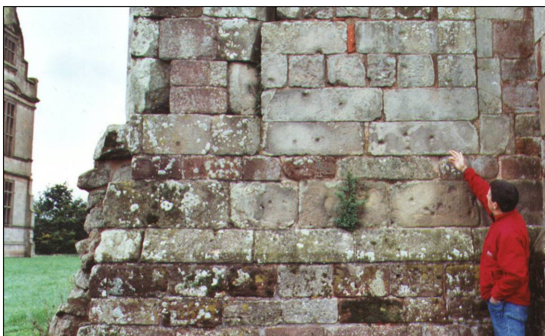
Figure 126: Section of wall at Moreton Corbett showing bullet impact scars
